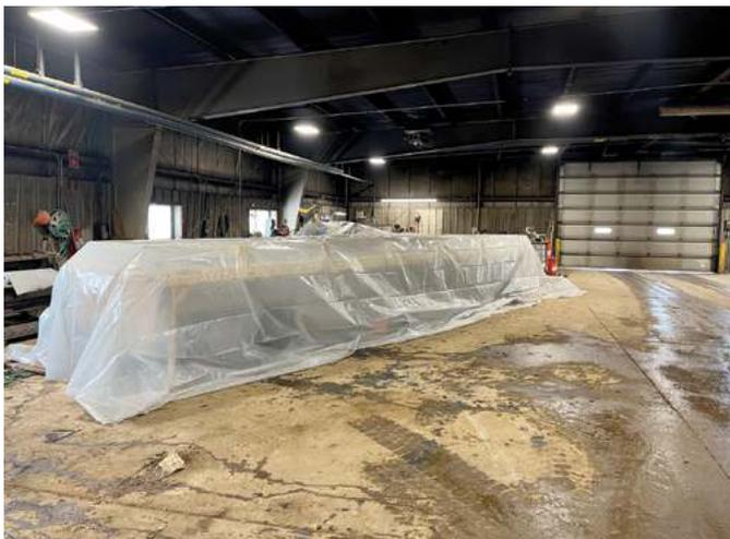
Fig. 9: Composite steel/UHPC girder covered in plastic sheet with heat source to promote curing of UHPC
