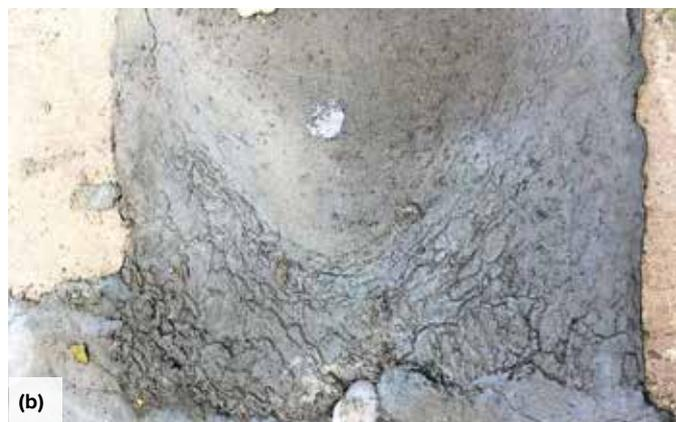
Fig. 5: Field placement after 1 day: (a) view of a UHPC connection; and (b) shrinkage cracks visible on the surface
